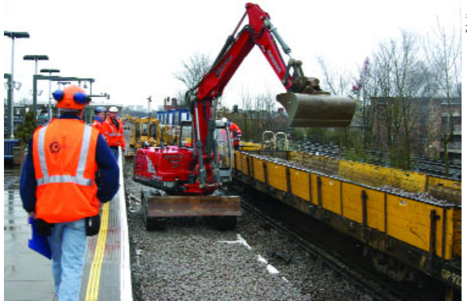
Enhanced track renewal at Kilburn on the Jubilee line.
