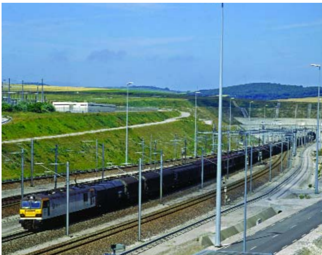
High access charges are deterring some rail freight operators from using the Channel Tunnel.
